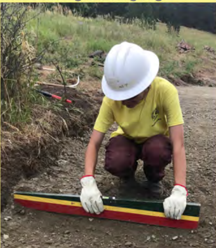
Ali checking the outslope using a trail gauge
