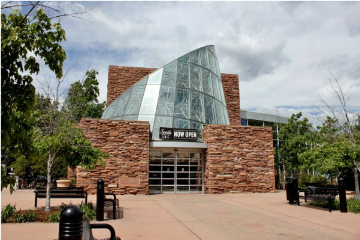
Example of a Public Building Utilizing a Pronounced Entry as a Wayfinding Feature
