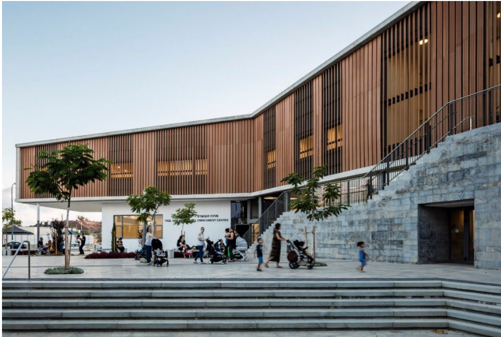
Example of a Public Building Framing the Adjacent Public Open Space
