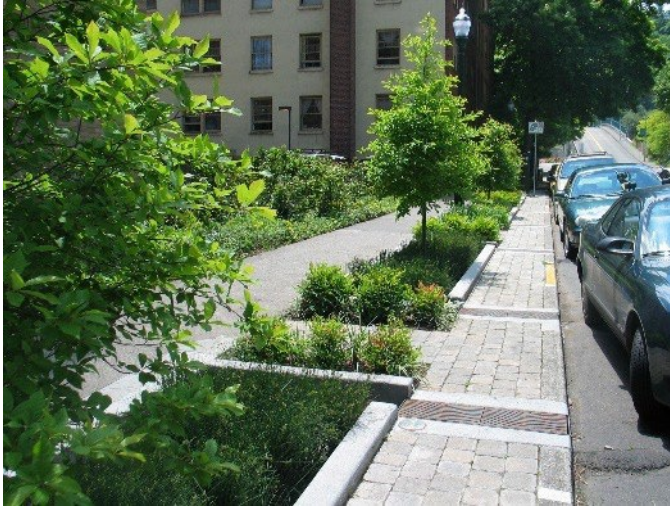
Example of Green Infrastructure Infiltration Planter
