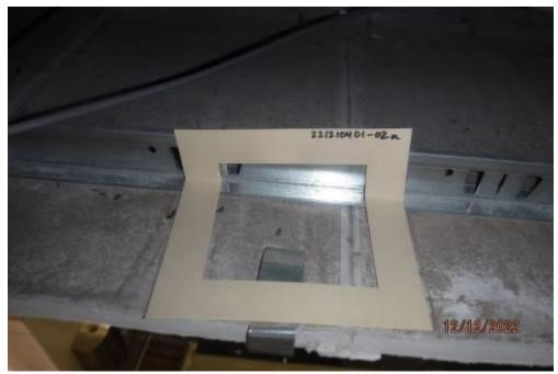
The main level women's restroom ducts and surfaces contained meth in excess of the decontamination criteria.
