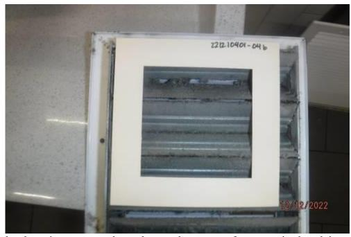
The upper level men's restroom exhaust ducts and contact surfaces contained meth in excess of the decontamination criteria.
