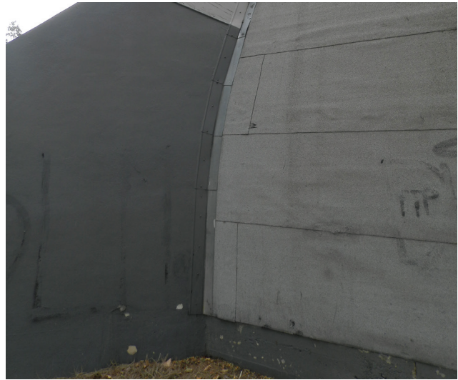
Figure 1-17. Rolled asphalt roofing. Note the blistering at the lower portion of the roof, 2020 (source: Ratio)
