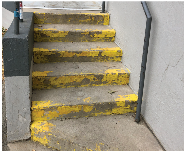
Figure 1-23. Concrete stairs. Note the yellow safety nosing paint condition is poor, 2020 (source: Ratio)
