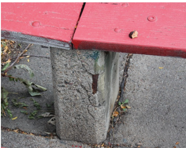
Figure 1-26. Spalling at pedestal of Amphitheater Seating, 2020 (source: Ratio)
