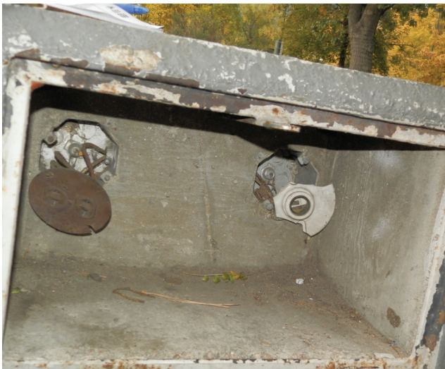
Figure 1-22. Interior view of lighting and power bollards. Note the cracking concrete forms, rusted and broken cover plates, as well as missing components, 2020 (source: Ratio)
