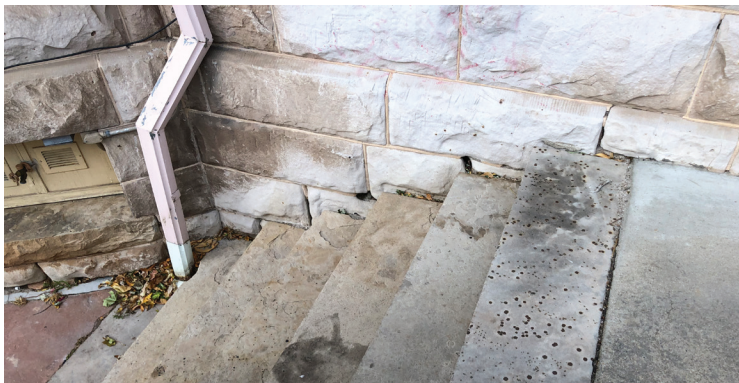
Figure 1-16. Stone damage at stair, 2020 (source: Ratio)
