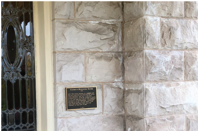
Figure 1-14. Efflorescence west of main entry, 2020 (source: Ratio)
