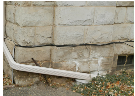
Figure 1-17. Stone damage at gutter, 2020 (source: Ratio)
