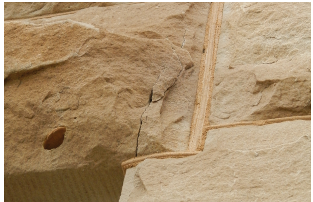
Figure 1-15. Cracked header, 2020 (source: Ratio)
