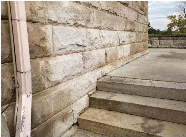
Figure 1-65. Erosion of stone at locations of graffiti removal, 2020 (source: JVA)
