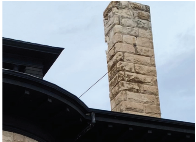
Figure 1-66. Deteriorated and loose stone at chimney
