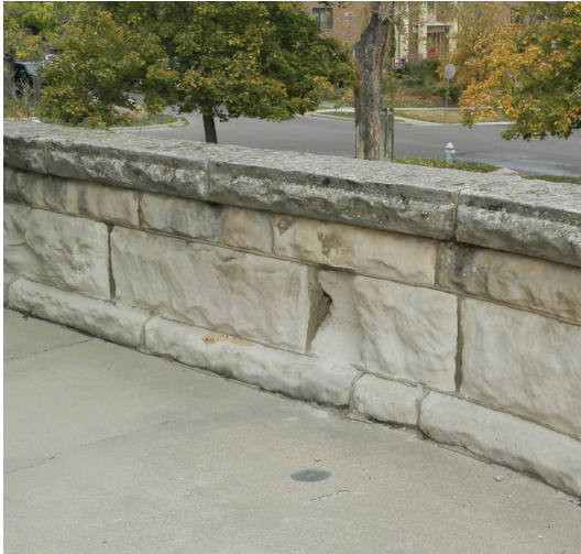
Figure 1-10. Stone damage at the interior porch wall, 2020 (source: Ratio)
