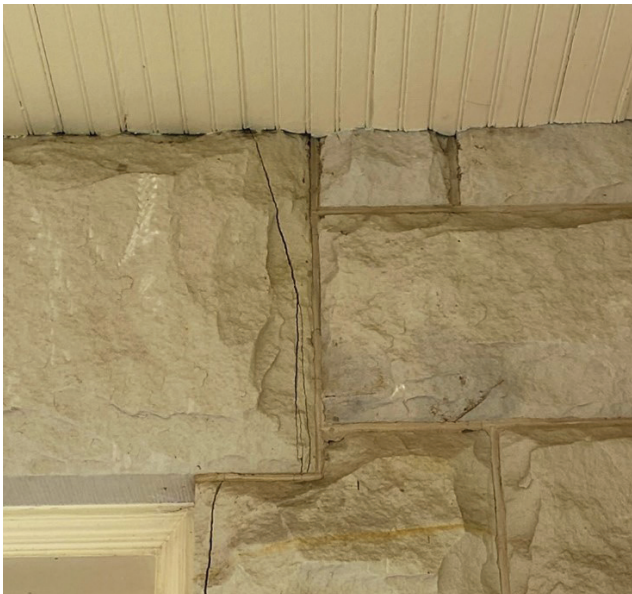
Figure 1-67. Thermal related cracking at door jamb, 2020 (source: JVA)
