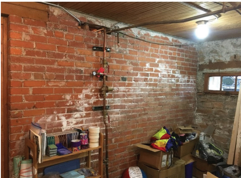
Figure 1-64. Efflorescence on basement walls, 2020 (source: JVA)
