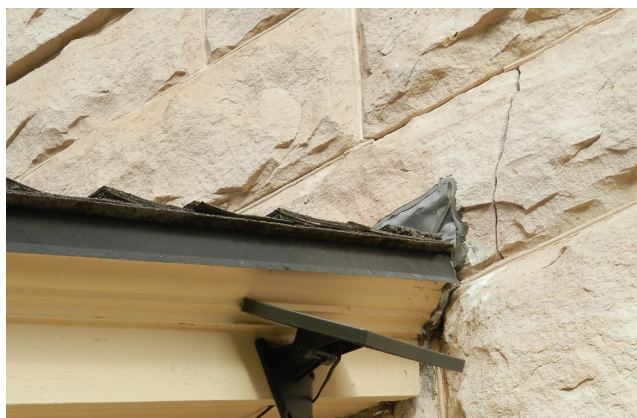
Figure 1-18. Cracked stone, 2020 (source: Ratio)
