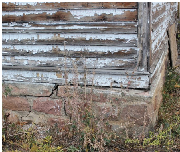
Figure 1-23. Southwest corner foundation settlement, 2020 (source: JVA)
