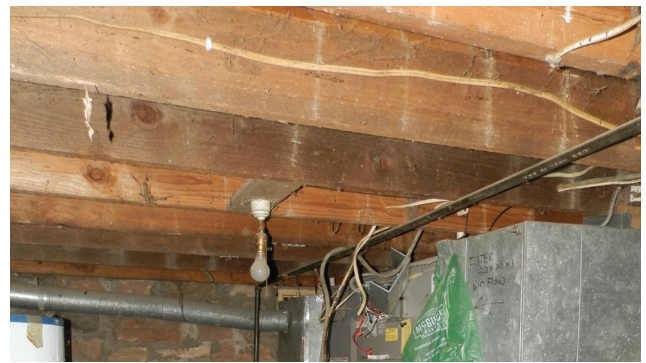
Figure 1-15. Main floor framing from basement, 2020 (source: Ratio)
