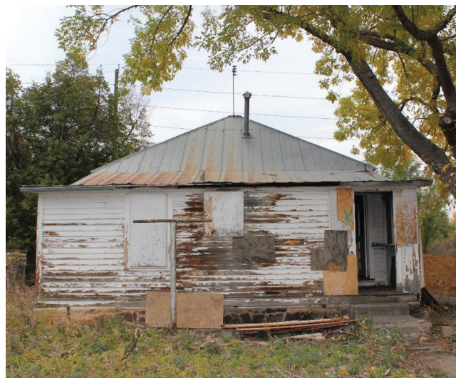
Figure 1-25. Back of Roney House, note rusted metal roof, 2020 (source: JVA)
