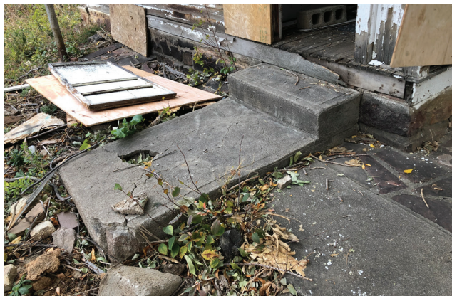
Figure 1-6. Damaged concrete sidewalk, 2020 (source: Ratio)
