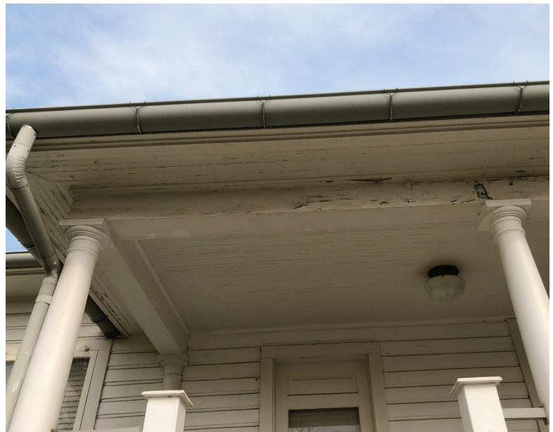
Figure 1-9. Wood porch framing roof supports, 2020 (source: Ratio)
