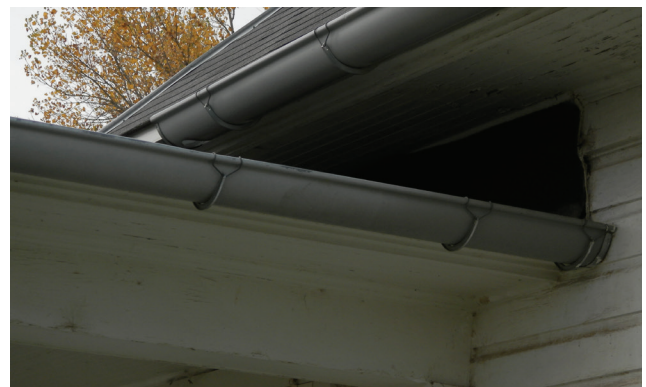
Figure 1-18. Half-round gutters, 2020 (source: Ratio)
