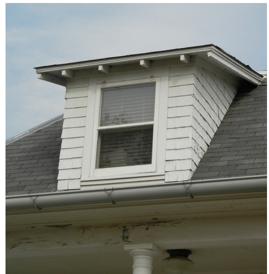
Figure 1-16. Wood shingle dormers, 2020 (source: Ratio)
