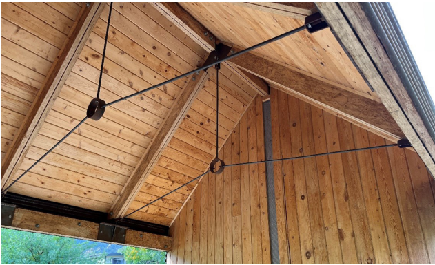
Figure 1-31. Typical roof framing of Volunteer Shed, 2022 (source: JVA)
