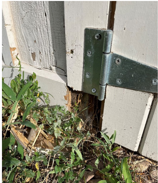
Figure 1-28. Broken trim at the west jamb of the south door, 2022 (source: JVA)
