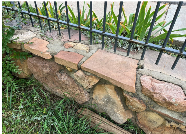
Figure 1-19. Typical stone masonry site wall around the east and north sides of the perimeter of the Columbia Cemetery, 2022 (source: JVA)
