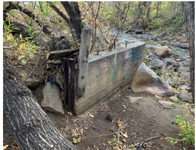
Figure 1-7. Concrete dam and headgate (source: Mundus Bishop)
