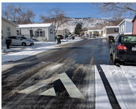
Through bilingual community engagement with the residents of Boulder Meadows and a strong collaboration with the Transportation Advisory Board, installed 17 speed humps in the neighborhood
