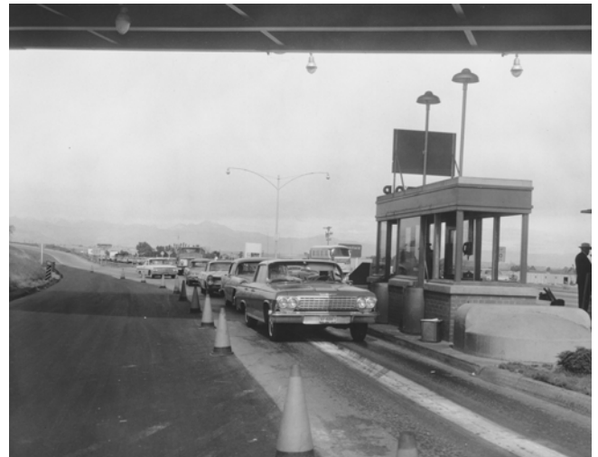
Figure 23 - The toll station at Broomfield along the Denver-Boulder Turnpike. photo, Boulder Daily Camera.
