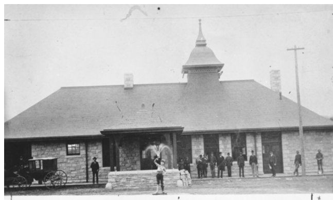
Figure 8 - The Depot at Fourteen and Water Streets, WCTU fountain in front. photo A.A. Paddock Collection.
