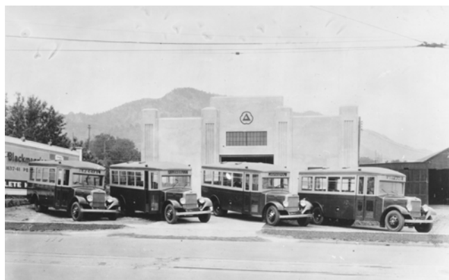
Figure 15 - Boulder's first bus system in its entirety, June 1931. Snow photo, Western Historical Collections, University of Colorado at Boulder
