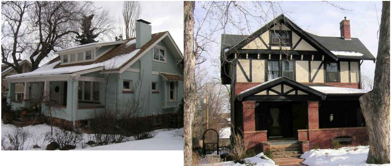
Figure 1-1. Historically contributing buildings located in designated historic districts, each of these houses had energy audits done in the winter of 2006-07. A number of opportunities were discovered for cost-effective energy-related retrofits in each house that will not affect their architectural or historic integrity.
