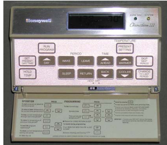
Figure 2-12. Electronic thermostats can save energy while preserving comfort.
