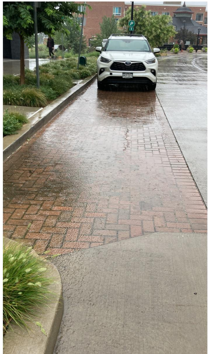
*Permeable pavement system along Junction Place*
