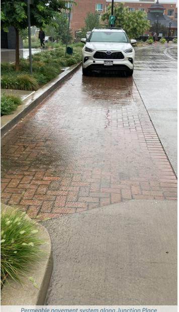
Permeable pavement system along Junction Place
