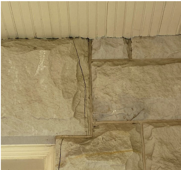
Figure 1-67. Thermal related cracking at header, 2020 (source: JVA)
