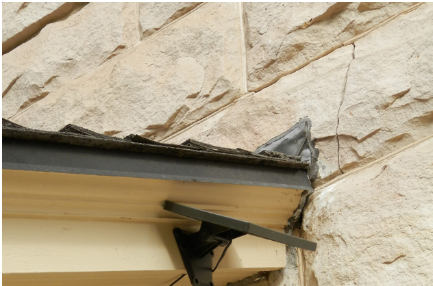
Figure 1-18. Cracked stone, 2020 (source: Ratio)
