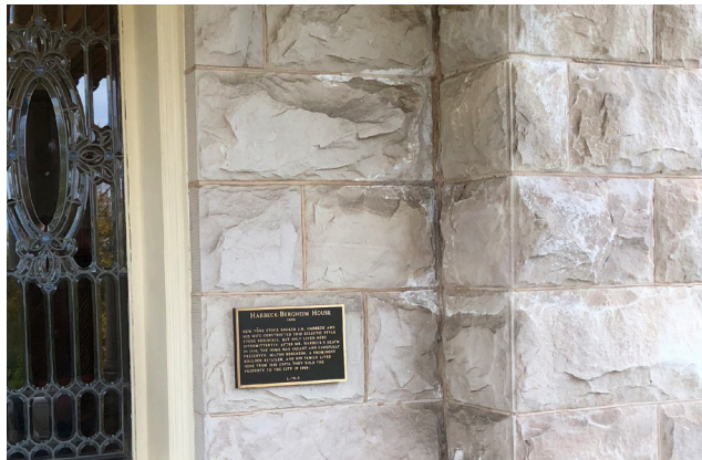
Figure 1-14. Efflorescence west of main entry, 2020 (source: Ratio)
