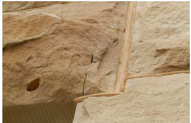
Figure 1-15. Cracked header, 2020 (source: Ratio)
