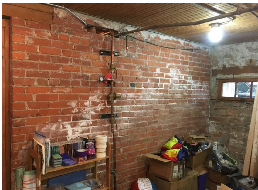
Figure 1-64. Efflorescence on basement walls, 2020 (source: JVA)
