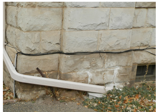
Figure 1-17. Stone damage at gutter, 2020 (source: Ratio)
