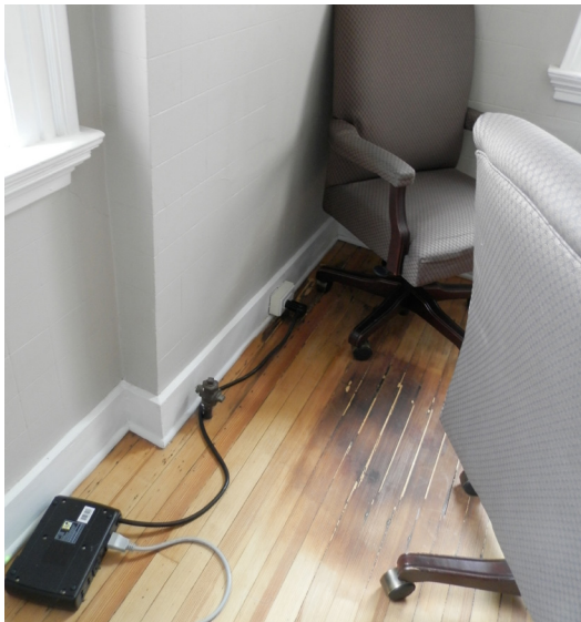
Figure 1-76. Second floor wood floor damage, 2020 (source: Ratio)
