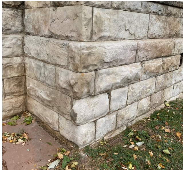
Figure 1-68. Erosion of stone near grade and lichen growth at coping, 2020 (source: JVA)
