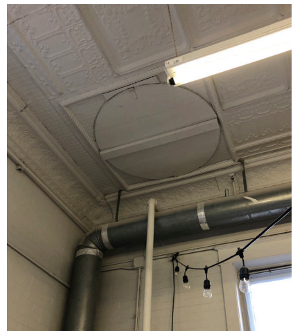
Figure 1-21. Original fire pole location, 2020 (source: Ratio)
