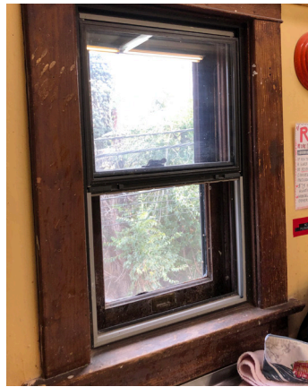
Figure 1-12. Upper level window with interior storm, 2020 (source: Ratio)
