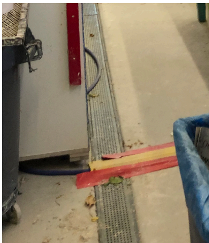
Figure 1-4. Linear floor drain, 2020 (source: Ratio)
