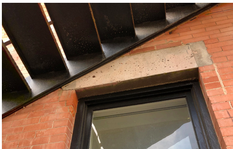
Figure 1-10. Lintel below exterior stair, 2020 (source: Ratio)
