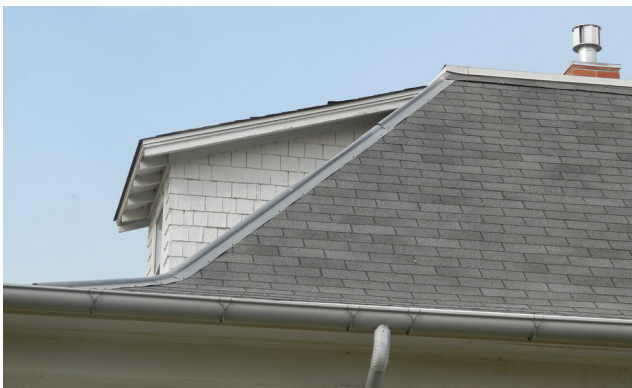
Figure 1-17. Asphalt shingle roof, 2020 (source: Ratio)
