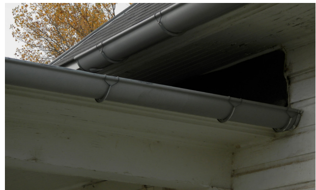
Figure 1-18. Half-round gutters, 2020 (source: Ratio)
