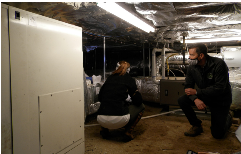
Figure 1-21. Swamp cooler and furnace in the crawl space, 2020 (source: Ratio)
