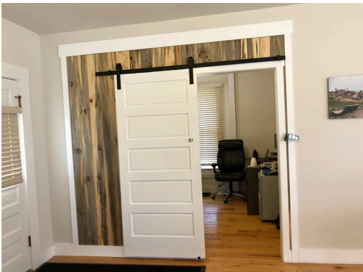
Figure 1-15. Sliding barn door and infill wall, 2020 (source: Ratio)
