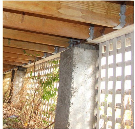
Figure 1-24. Porch piers wrapped in coating, 2020 (source: JVA)
