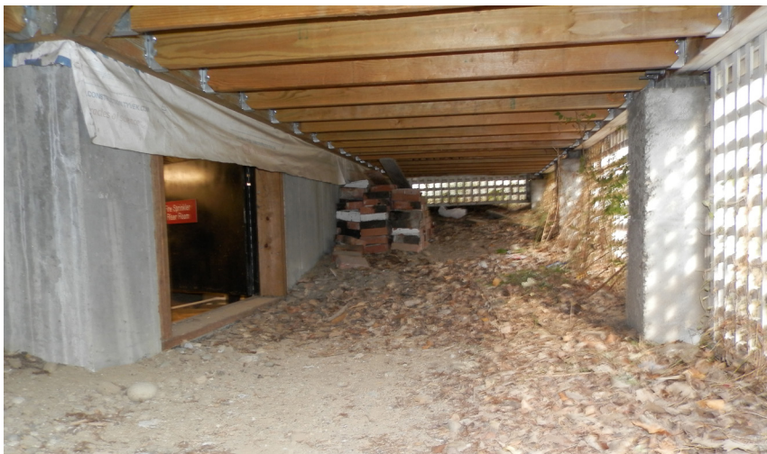
Figure 1-6. Porch and building foundations, 2020 (source: Ratio)
