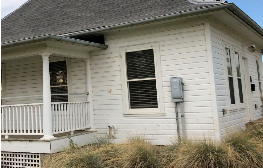
Figure 1-10. Wood siding, 2020 (source: Ratio)
