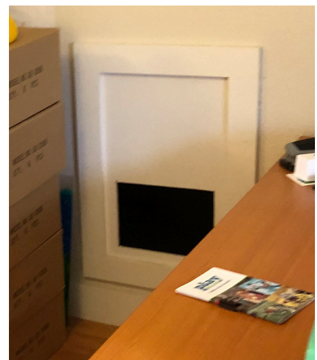
Figure 1-22. Attic access panel, 2020 (source: Ratio)
