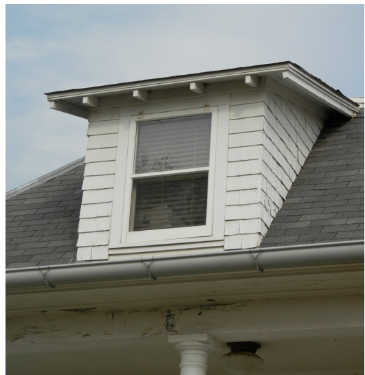
Figure 1-16. Wood shingle dormers, 2020 (source: Ratio)
