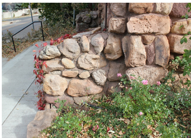
Figure 1-25. Differential settlement crack at northwest buttress, 2020 (source: JVA)
