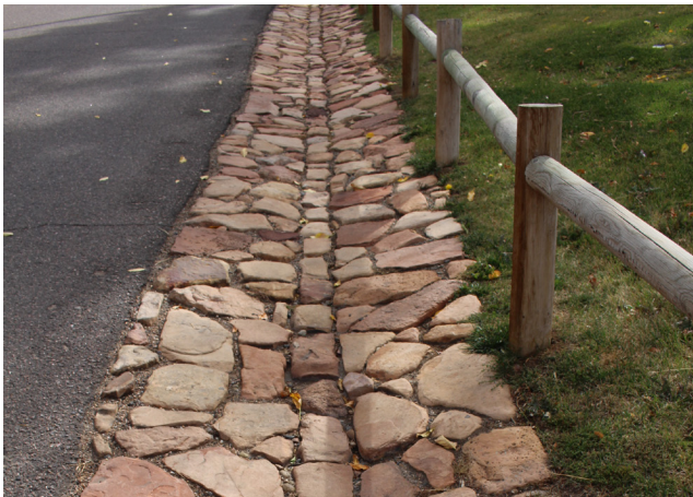
Figure 1-39. Stone gutters built using in-kind compatible materials on Sumac Drive, 2020 (source: Mundus Bishop)
