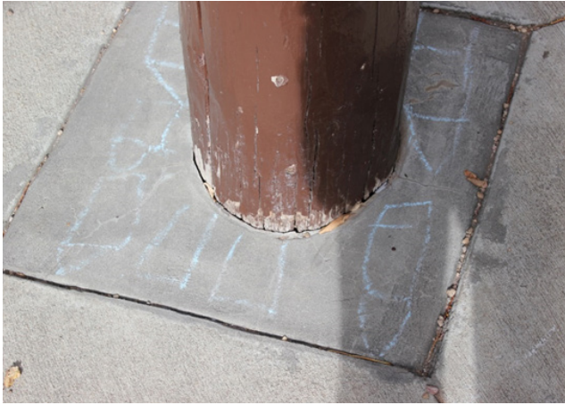
Figure 1-18. Decay at base of timber post, 2020 (source: JVA)
