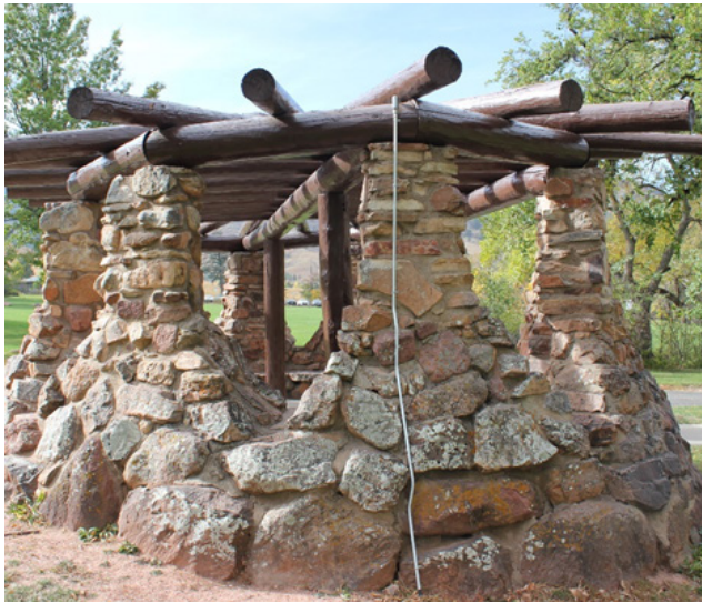
Figure 1-16. The Arbor, note lichen growth and eroded mortar joints, 2020 (source: JVA)
