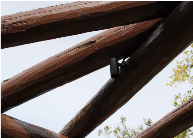
Figure 1-20. Interior lights hidden in timbers, 2020 (source: JVA)
