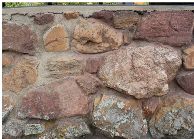
Figure 1-24. Repair mortar – note red color and separation cracks, 2020 (source: JVA)
