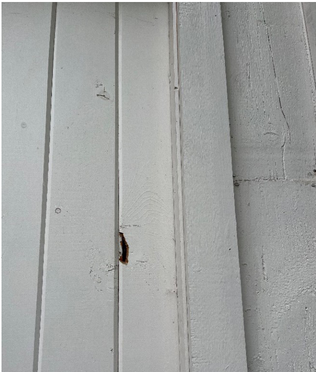
Figure 1-27. Impact damage on a panel in the wood door of the building, 2022 (source: JVA)
