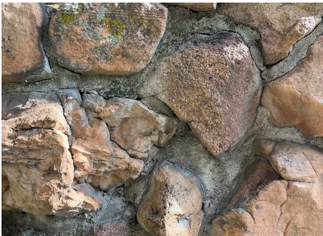
Figure 1-18. Some of the sandstone units are slightly eroding as evidenced by their rounded edges on the Pioneer Gateway, 2022 (source: JVA)
