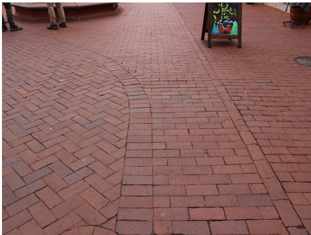
Figure 1-23. Brick paving with curving central herringbone pattern at 1100 Block, 2020 (source: Mundus Bishop)
