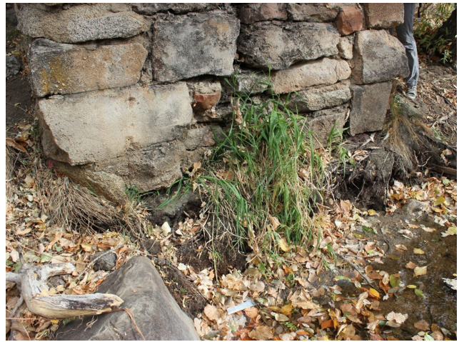
Figure 1-16. Base of north pylon. Note the scour at the creek bank's edge, 2020 (source: JVA)
