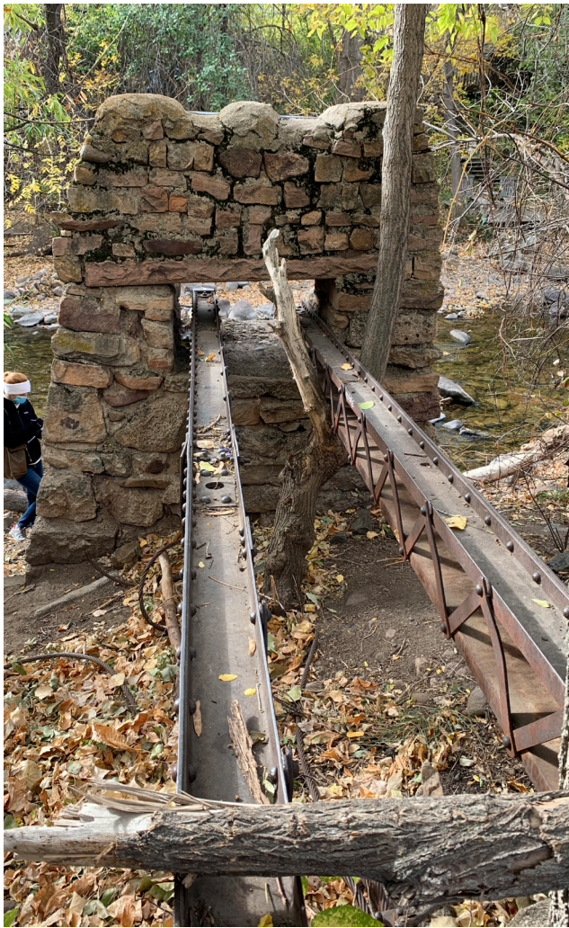
Figure 1-6. North pylon with steel support girder, 2020 (source: Mundus Bishop)
