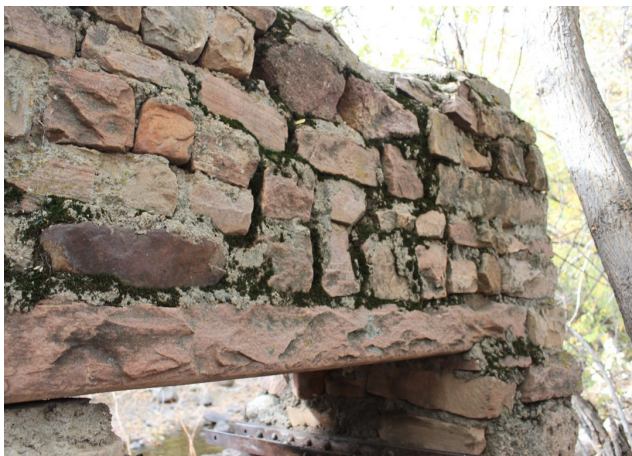
Figure 1-13. Biogrowth and areas of missing mortar, 2020 (source: JVA)
