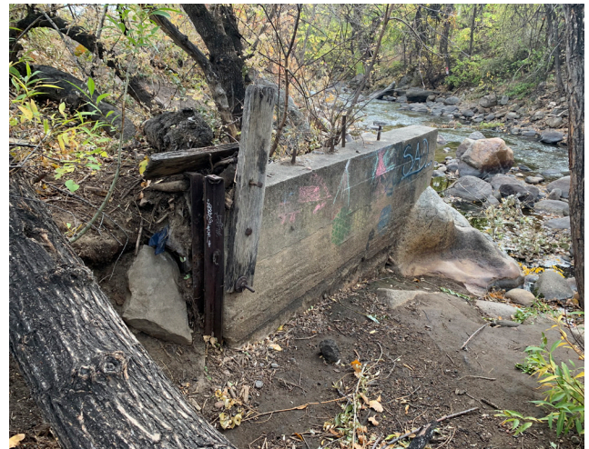
Figure 1-7. Concrete dam and headgate, recent and previous vandalism (source: Mundus Bishop)
