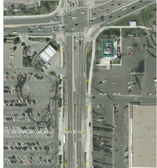
Figure 1: An aerial view of the Iris and 28th St. intersection. The LED pilot lights will be installed south of this intersection, indicated by the yellow circles.
