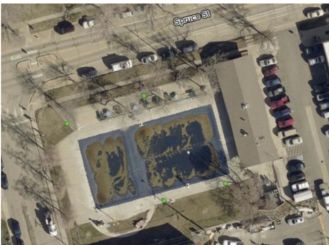
Figure 2: An aerial view of Spruce Pool. The LED pilot lights will be installed on the deck of the pool, indicated by the green circles, and are visible from the surrounding sidewalk.
