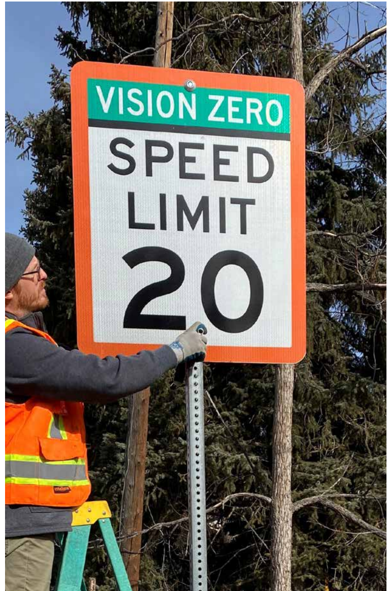
Vision Zero Sign Installation
