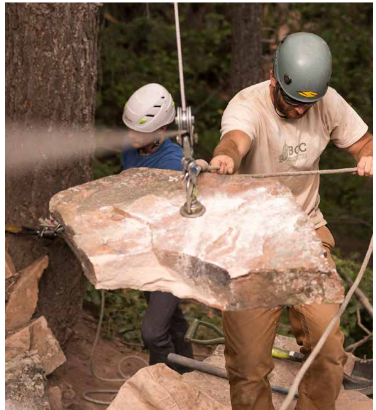
Trail Work on Boulder Open Space
