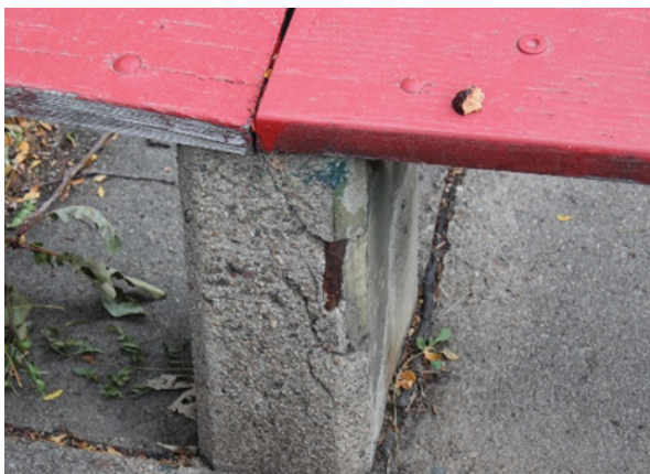
Figure 1-26. Spalling at pedestal of Amphitheater Seating, 2020 (source: Ratio)
