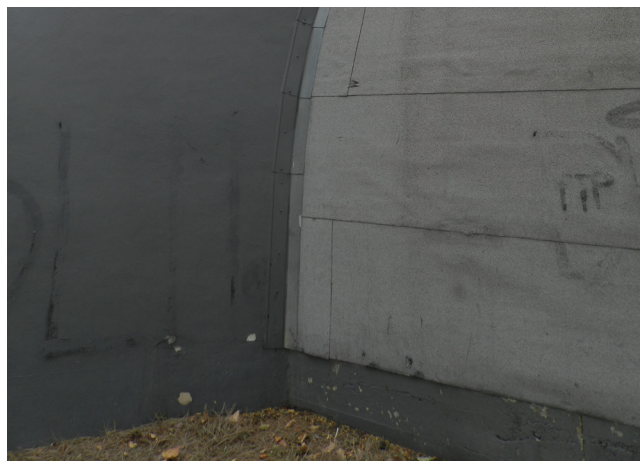
Figure 1-17. Rolled asphalt roofing. Note the blistering at the lower portion of the roof, 2020 (source: Ratio)
