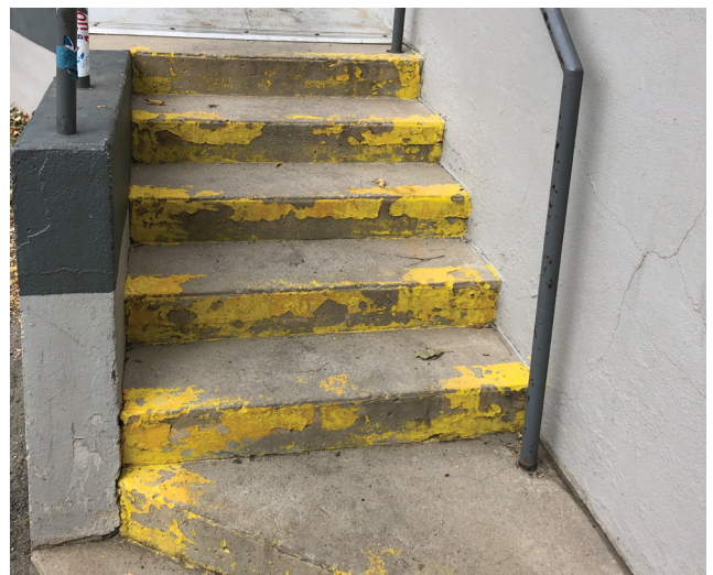
Figure 1-20. Concrete stairs. Note the yellow safety nosing paint condition is poor, 2020 (source: Ratio)
