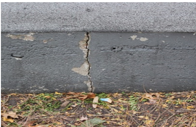
Figure 1-24. Vertical foundation crack on the east side, 2020 (source: Ratio and JVA)
