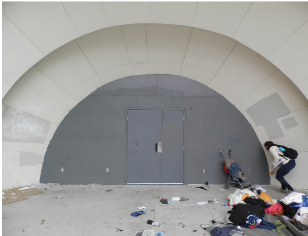
Figure 1-22. Exterior plywood finish panels, 2020 (source: Ratio)
