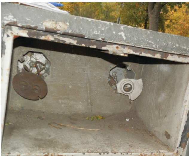
Figure 1-18. Interior view of lighting and power bollards. Note the cracking concrete forms, rusted and broken cover plates, as well as missing components, 2020 (source: Ratio)
