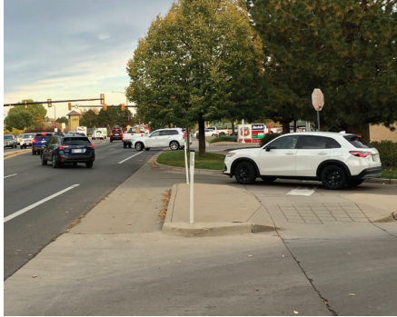
Northern driveway for Safeway shopping center
