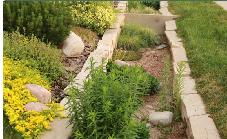
Bioretention area is protected by stone barriers to help indicate that the area should not be trafficked.
