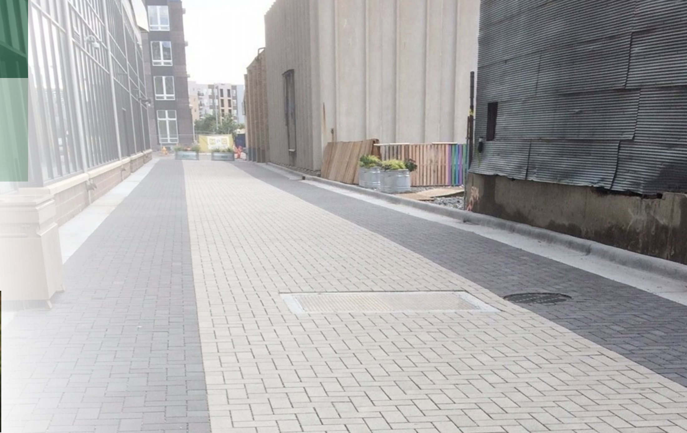
Example of permeable pavement adding visual interest and sense of place to a downtown area.
