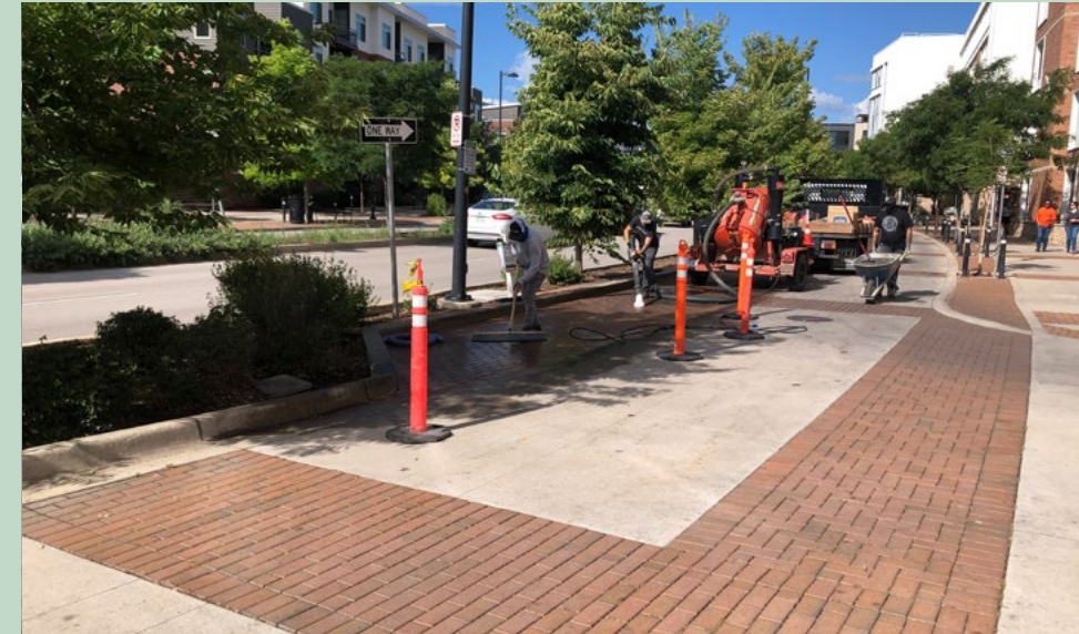
Maintenance on this permeable pavement system involved blocking of multiple paid parking spots and closing a small side street.
