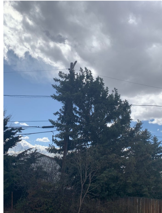
Tree fall into distribution cross-arm Arvada, CO
