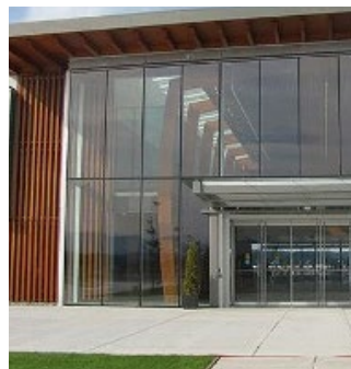
Glass Curtain Wall
