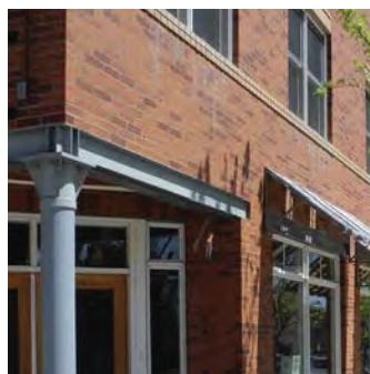
Brick with Metal Details
