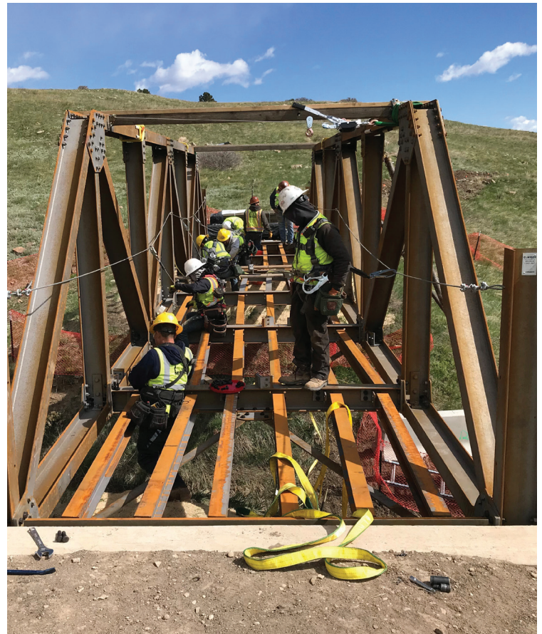
North Sky Trail Bridge Installation
