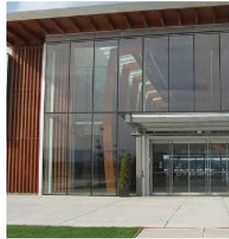
Glass Curtain Wall
