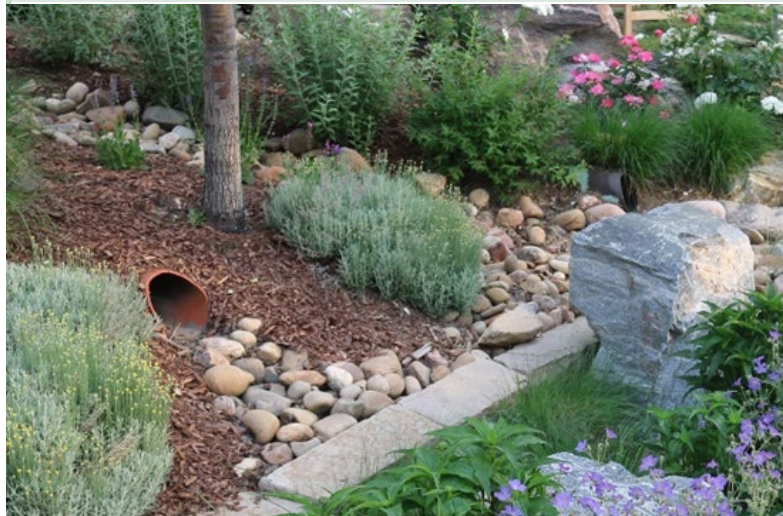
The inlet of this bioretention area is clean and free of debris, allowing runoff to enter the main treatment area.
