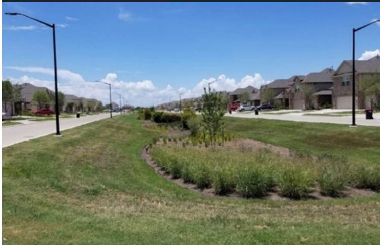
While there are no signs of vehicle or pedestrian traffic, adding informational signs about the bioretention area could help protect the SCM from intrusion and damage.
