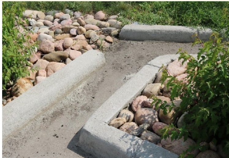
The inlet has sediment buildup, which could prevent the SCM from draining properly. The sediment should be removed with a shovel and disposed of.
