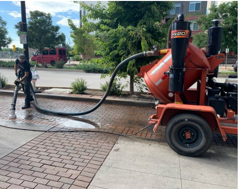
Using a pressure washer with a Ditch Witch FX20 Vacuum to dislodge material from the joint spaces.
