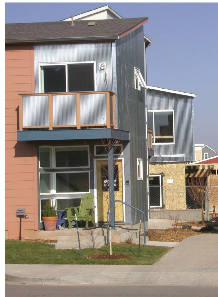
The Holiday neighborhood under construction in 2001 following the 1997 North Boulder Subcommunity Plan.
