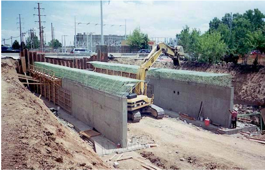
Drainage improvement project on Goose Creek at 28th Street, Boulder
