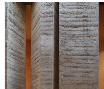
Rammed earth walls
