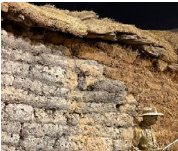
Sod wall fort construction
