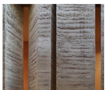
Rammed earth walls
