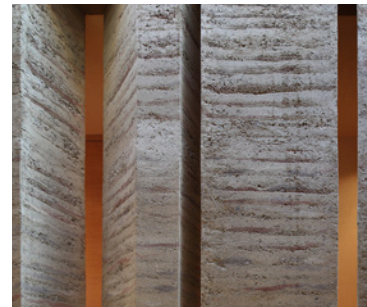
Rammed earth walls
