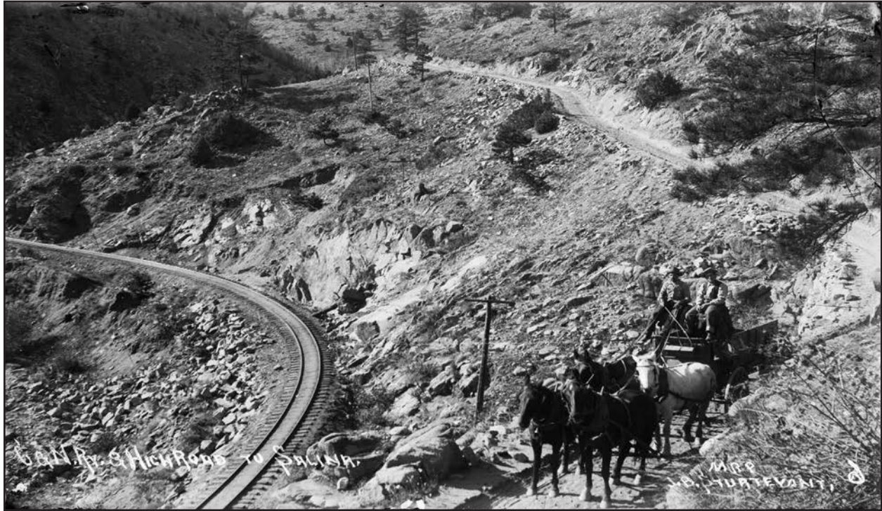
In Four Mile Canyon, below Salina, a "high-line road" was built well out of the path of future floods. This photo was likely taken in 1898, after the rebuilding of the narrow-gauge railroad track. Carnegie Branch Library for Local History, Boulder Historical Society collection S-2509
