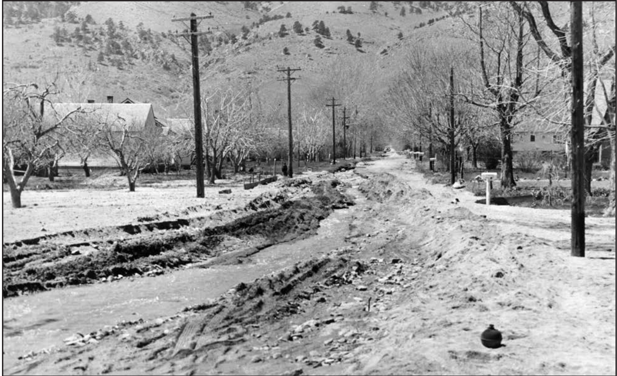
After debris blocked a bridge over Two Mile Creek, water rushed down Iris Avenue (formerly 9th Avenue) during the April 24, 1942 flood. Boulder County crews rushed to sandbag the creek at Broadway and divert the water into Farmers Ditch. Carnegie Branch Library for Local History, Boulder Historical Society collection, 225-4-31 #1
