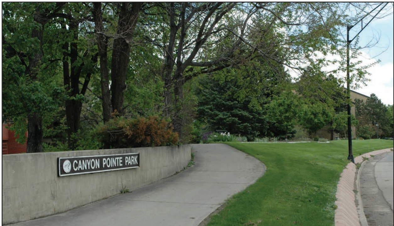
This area northeast of Canyon Boulevard and 6th Street was raised in 1978 to create a berm in order to protect a housing project from flooding. Author's photo, 2015
