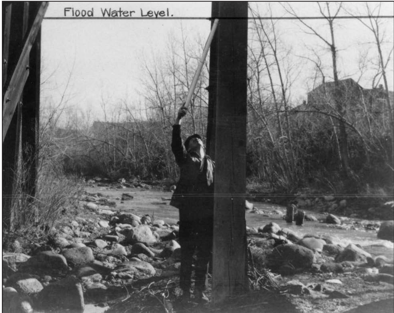
This photo was taken in 1911 below the railroad bridge that crossed Boulder Creek at 4th Street. The man in the photo is showing how high the flood waters got during the flood of 1894. (See Part II, Metcalf and Eddy Report.) Carnegie Branch Library for Local History, Boulder Historical Society collection, 225-3-27 #1
