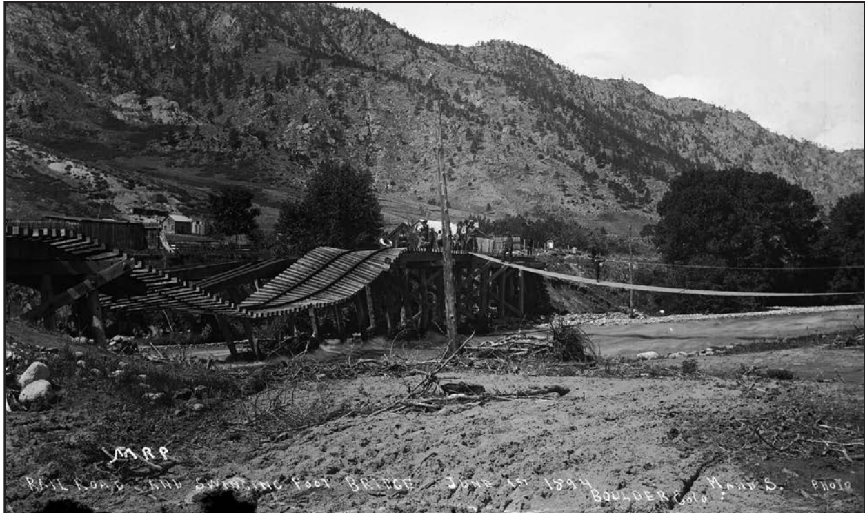
The railroad bridge over Boulder Creek, at 4th Street, looked like this after the 1894 flood. See page 21 for a later photo of the flood water level mark under this bridge. Carnegie Branch Library for Local History, Boulder Historical Society collection, S-1292 (715-2-23 #1)
