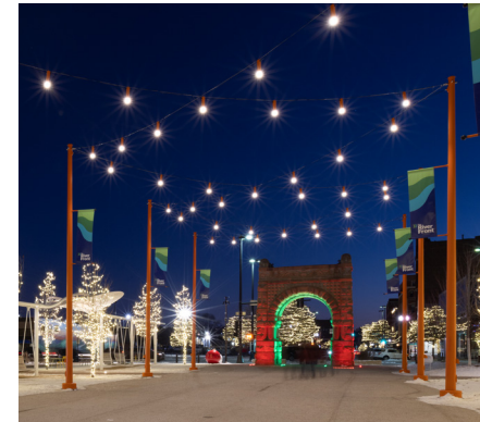
Lighting Pole - Promenade
