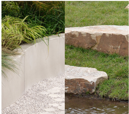
Site Wall (Concrete + Stone)
