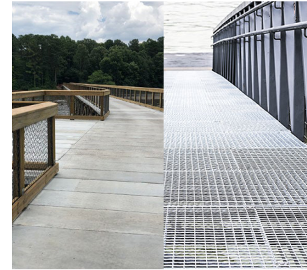
Boardwalk (Concrete, Metal)
