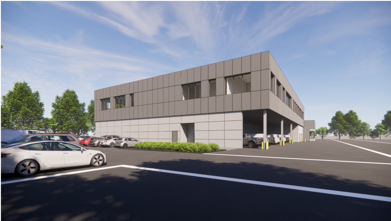
SERVICE CENTER - NORTHEAST
