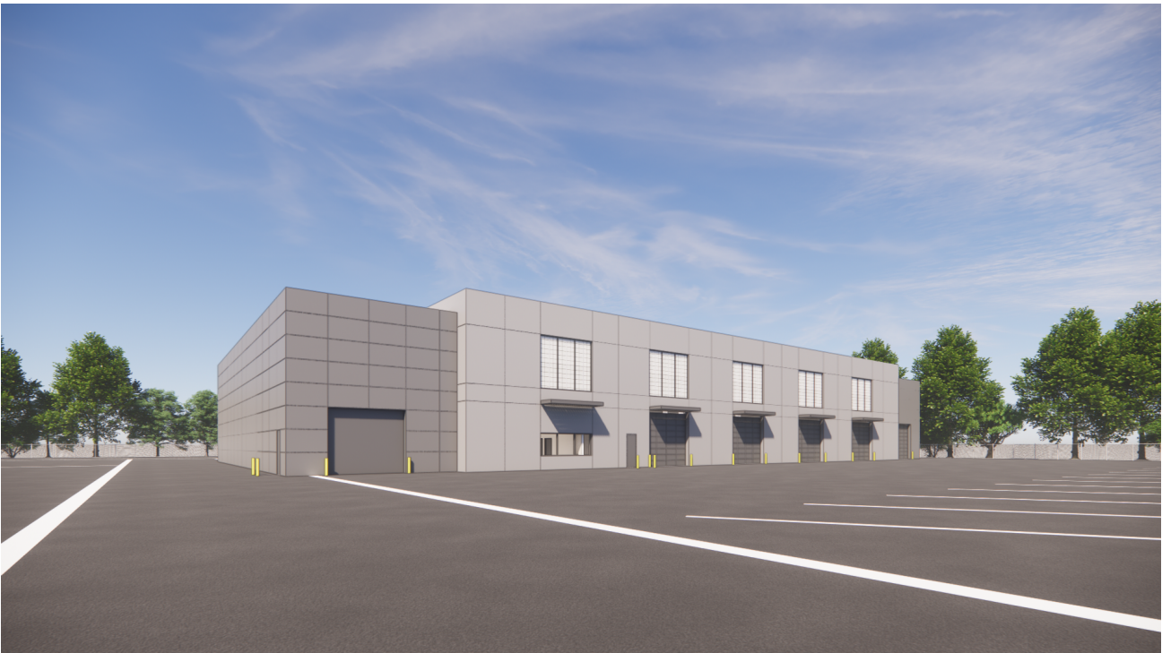
FLEET GARAGE - SOUTHWEST
