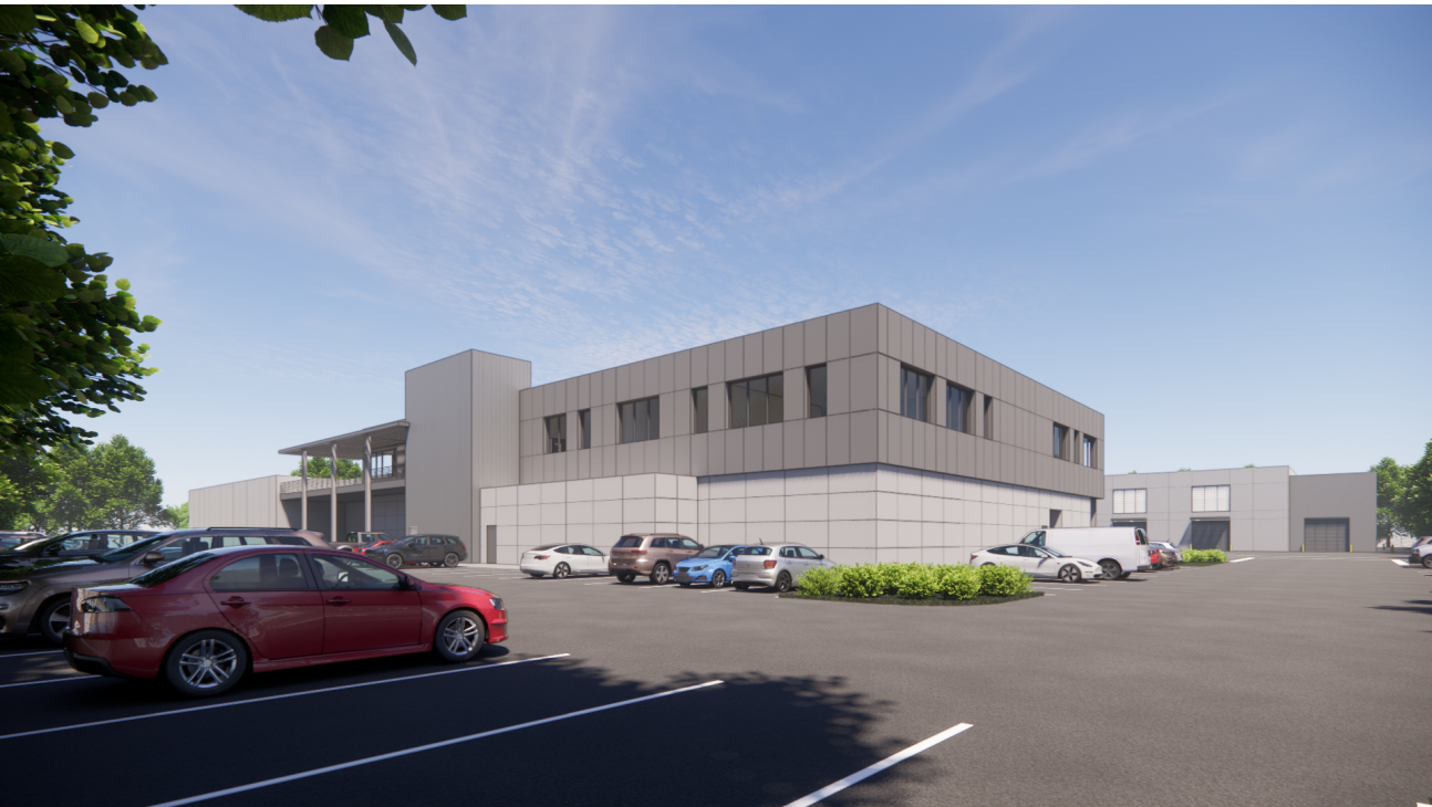
SERVICE CENTER - SOUTHEAST
