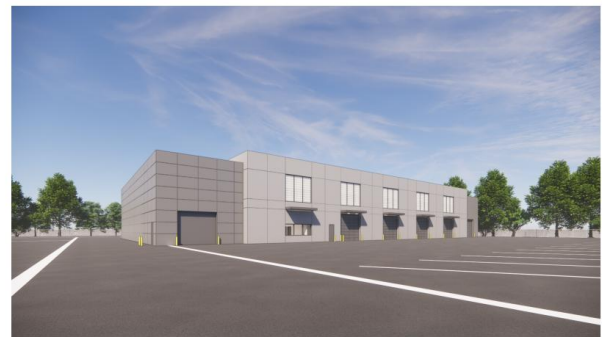
FLEET GARAGE - SOUTHWEST
