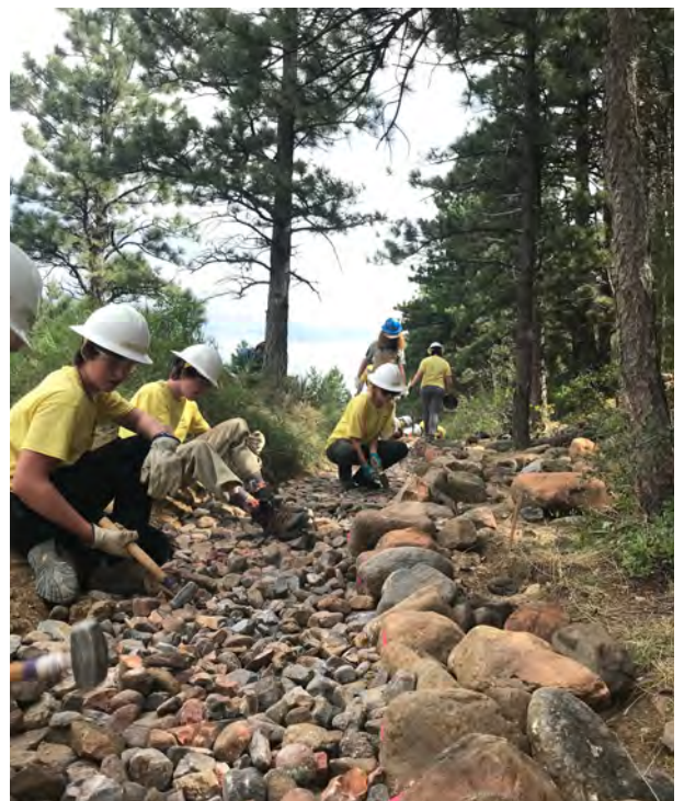
Below: Setting cobble on the turnpike on Doudy Draw.
