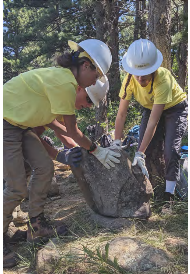
Rock work requires patience, teamwork, and good communication.
