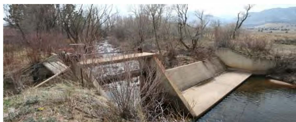
Ditch Diversion a Barrier to Fish Passage
