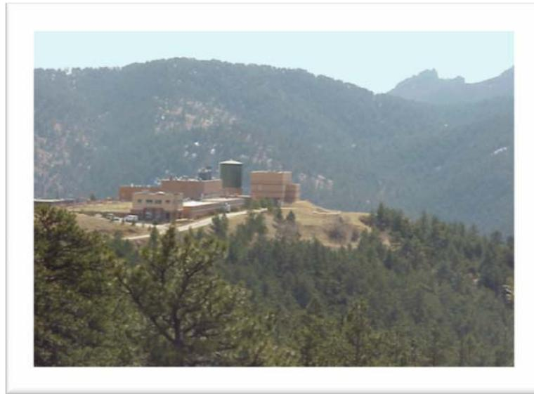
Betasso WTF was expanded to its present capacity in 1976. At about the time of the expansion, 50 MGD became widely accepted as the design capacity of the Betasso facility. However, hydraulic limitations and the need to limit flow into the filter beds to meet drinking water standards cause actual maximum facility capacity to be closer to 45 MGD<sup>154</sup>.
