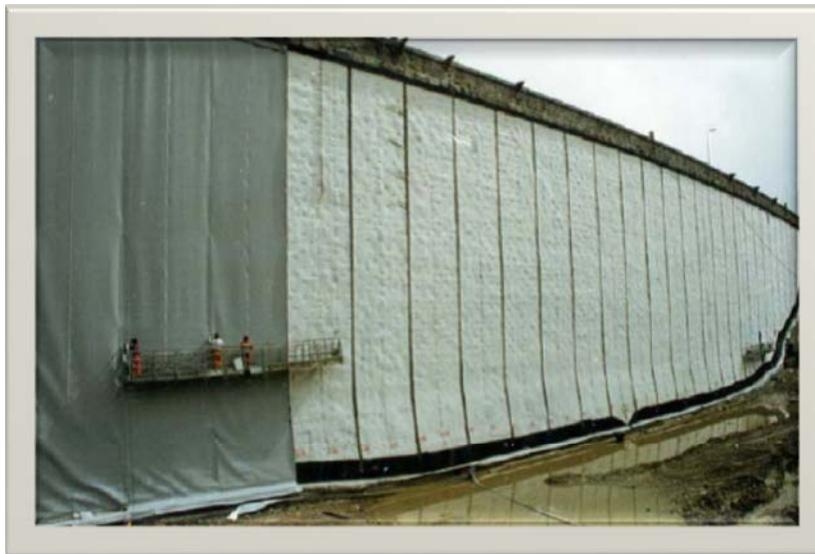
**ISLAND DAM (3)** - Damage to the dam crest wall and upstream face need immediate repair in order to prevent additional damage and to continue operation of the dam (Staff facilities tour, September 20, 2007). Island Dam is a very important facility. Despite its small storage volume, the water rights associated with Island Lake are very senior. Patches are recommended in five to seven locations near the high water mark.
