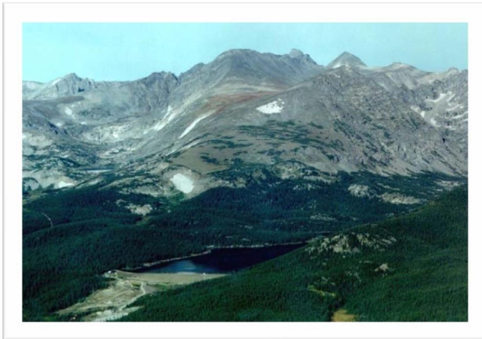
Silver Lake is formed by a 1,450-foot long earth fill embankment which is approximately 70 feet high at its maximum section. The dam was originally constructed by J. P. Maxwell for the Silver Lake Ditch Company in 1887 as a timber crib, rock fill dam<sup>84</sup>. The city acquired the reservoir in 1906<sup>85</sup> and did some repair work at that time. The dam was damaged by fire in 1910 and City Council
