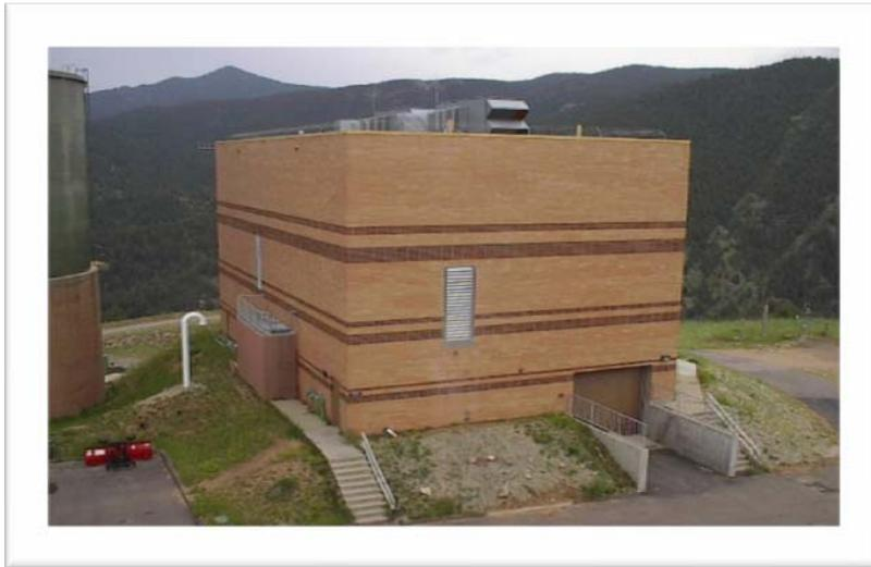
While the Betasso unit has a rated capacity of 3.2 MW, the plant currently can only achieve about 2.4 MW due to operating constraints in the Betasso Penstock. Replacement of the Betasso Penstock, scheduled for 2009, will allow Betasso Hydro to achieve its intended capacity and will increase hydropower revenue to the city.
