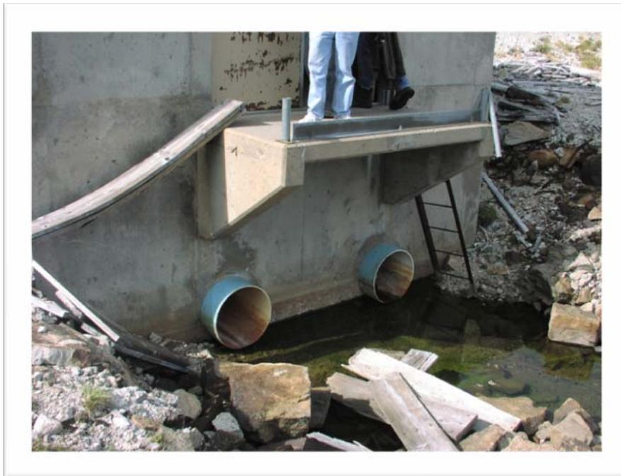
A structural inspection of Albion Dam was performed in 2002<sup>56</sup>. This inspection noted extensive spalling on the upstream lower half of the dam and excessive concrete deterioration along construction joints (see Figure 6-14 and Figure 6-15). A 1986 investigation<sup>57</sup> found that below the crest cap, the dam was mostly rubble for an estimated 10 feet in some areas. The ultimate conclusion
