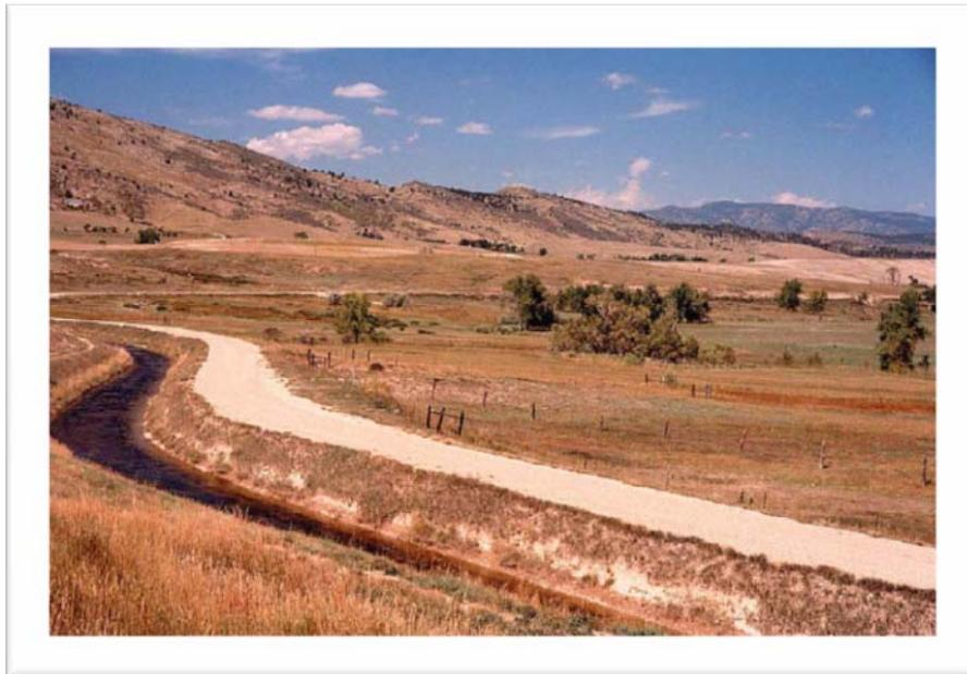
Canal operation is dictated primarily by the amount of demand for CBT deliveries for municipal and irrigation uses. The canal is typically out of service between November and April each year due to freezing.
