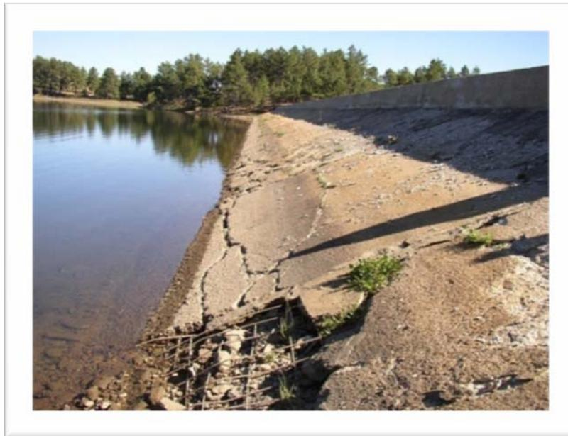
Seepage is evident downstream of the dam and is measured via a weir. Flows may bypass the seepage weir. Also, the piezometers may not be correctly located to measure the phreatic surface through the dam embankment. Woody shrubs growing on the upper downstream face of the dam could indicate a high phreatic surface. The upstream dam face shows severe spalling and cracking at and below the normal water level<sup>86</sup>.
