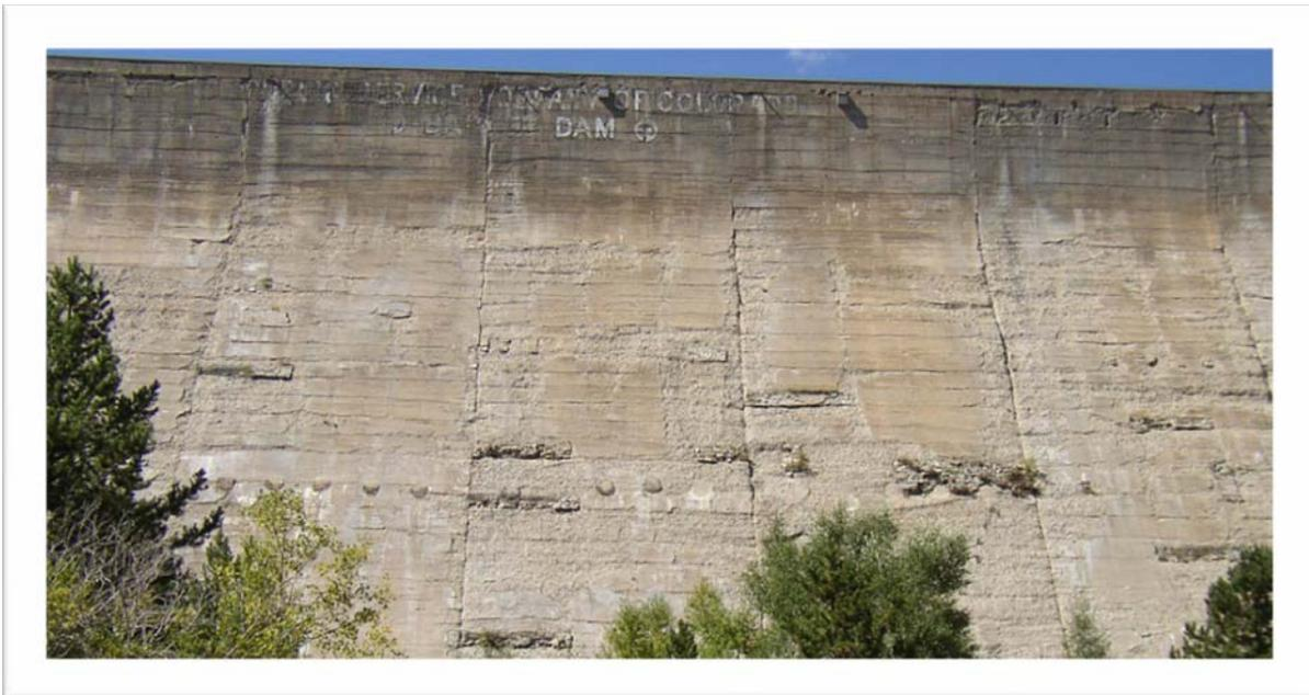
Spalling of the anchor head concrete caps (see Figure 6-20) was observed on the dam crest during the 2007 site visit. This spalling is not likely to affect dam function or stability in the near future. However, as spalling worsens, the anchors could potentially deteriorate.
