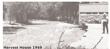
Boulder Creek flood - 1969
