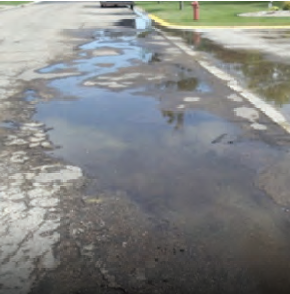
Poor Drainage
