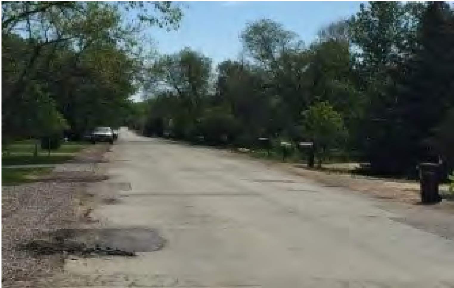
Deteriorating Pavement
