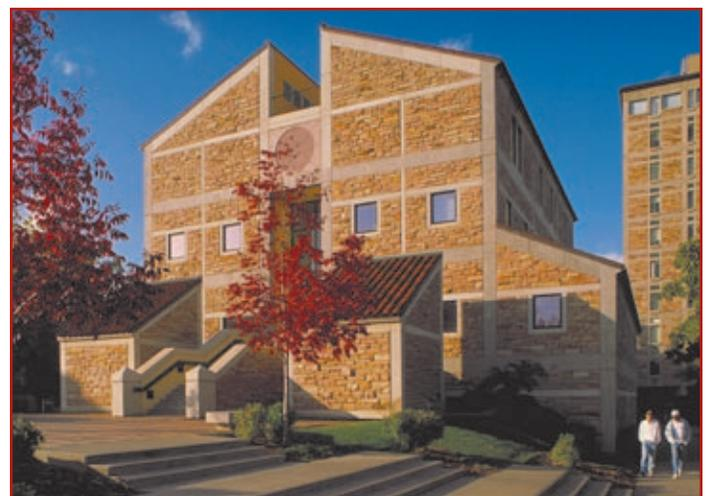
Two shed structures flanking the entry to the Joint Institute for Laboratory Astrophysics (JILA) addition contains a heat pump for the Power House in one, and a transformer in the other. Innovative solutions keep faith with quality campus architecture.
