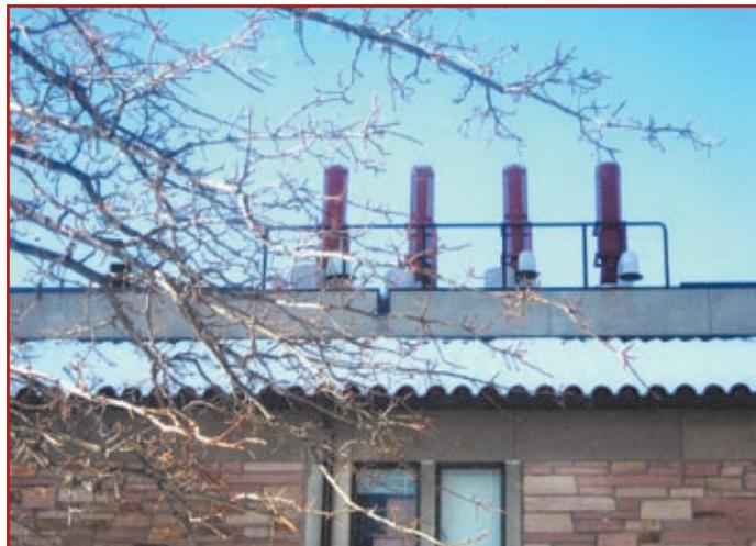
Roof equipment is ganged together and painted according to campus standard for such elements.
