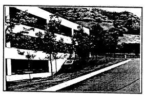
5.2.6 WHERE FEASIBLE, CREATE SLOP-ING TOPOGRAPHY TO PROVIDE GRADE ACCESS TO EACH LEVEL OF PARKING DECK.
