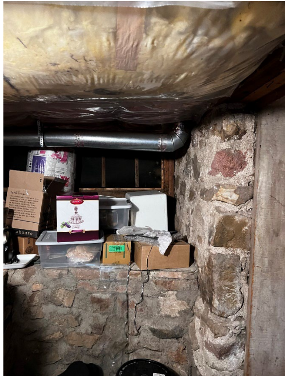
Existing basement with rumble stone foundation.
