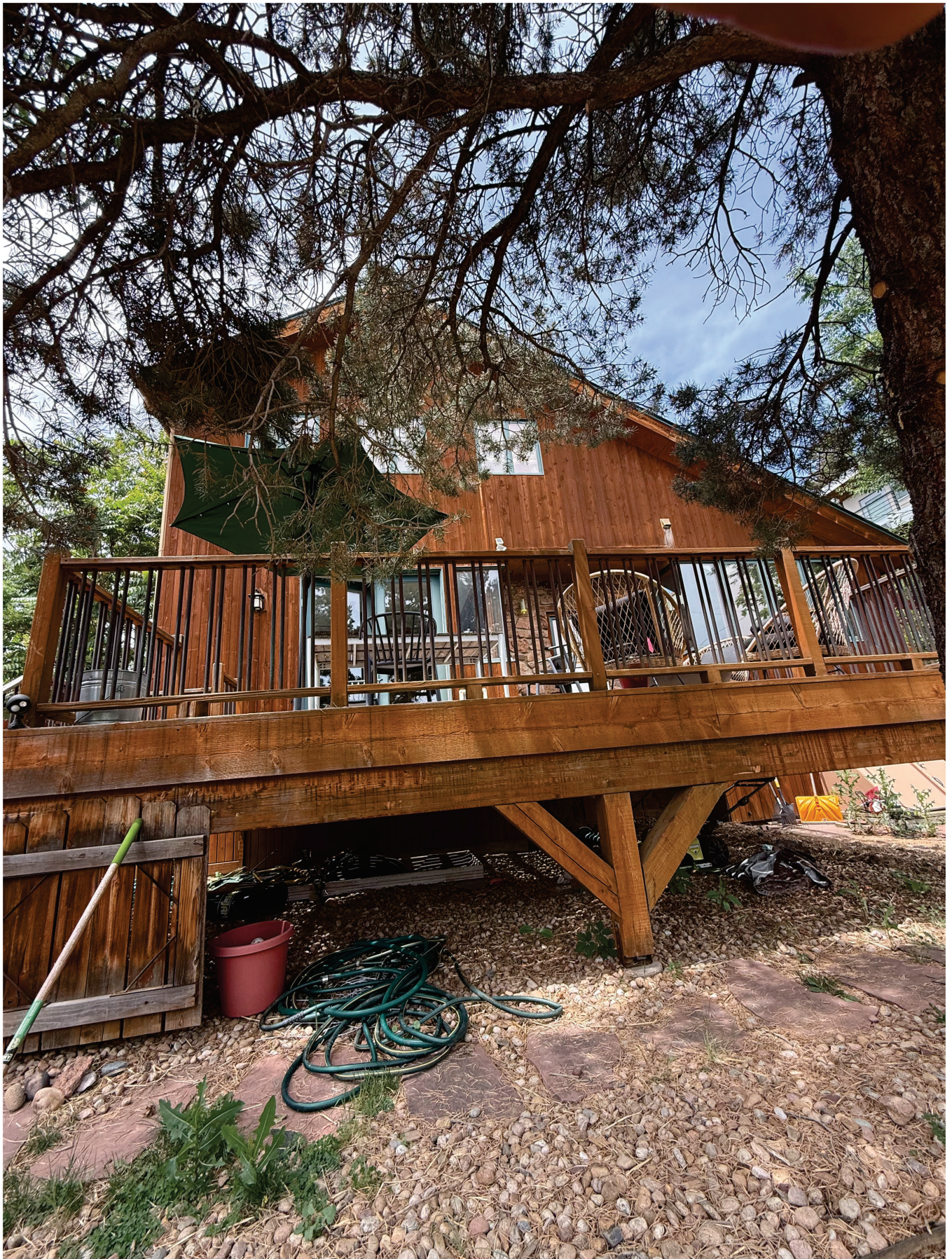
2910 5th St Existing Deck
