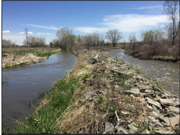
THE HOWELL DITCH (LEFT) RUNS NEXT TO BOULDER CREEK (RIGHT). DITCHES TYPICALLY HAVE FLATTER SLOPES AND SLOWER FLOWS THAN NATURAL DRAINAGES.
