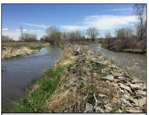
THE HOWELL DITCH (LEFT) RUNS NEXT TO BOULDER CREEK (RIGHT). DITCHES TYPICALLY HAVE FLATTER SLOPES AND SLOWER FLOWS THAN NATURAL DRAINAGES.
