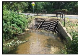
TRASH RACKS COLLECT DEBRIS FLOATING DOWN THE DITCH. THEY NEED TO BE CLEANED REGULARLY BY THE DITCH COMPANY
