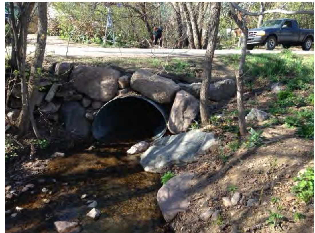
Post Flood Repair
