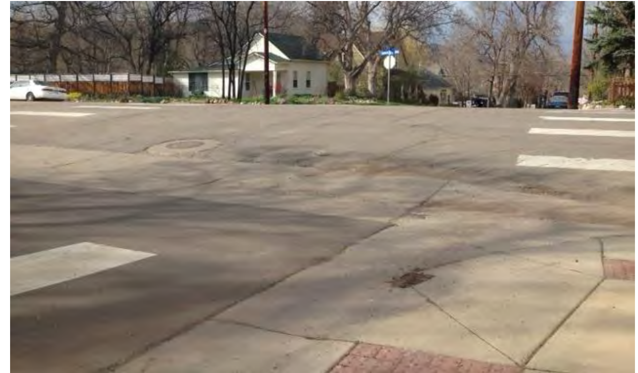
Existing Roadway Crown of University Ave. at 7 th St.
