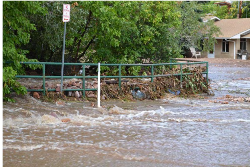
Sept. 2013 Flood Damage
