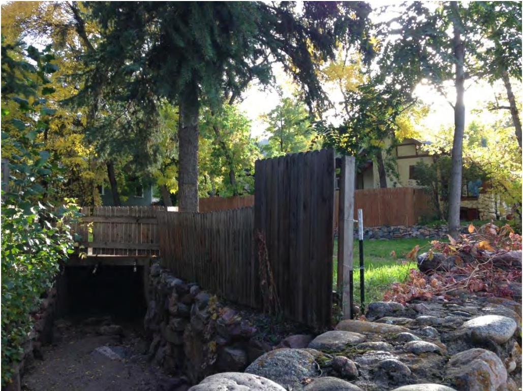
810 Marine After Deconstruction
