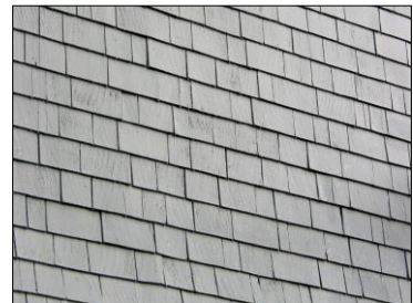
Historic materials such as wood siding, stone, brick and dimensional shingles help establish human scale.
