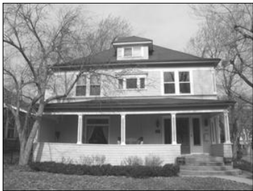
Foursquare Mayall-Pickett House Highland Avenue
