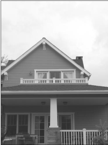
3.2.2 This rear roof deck is appropriately integrated into the roof.
