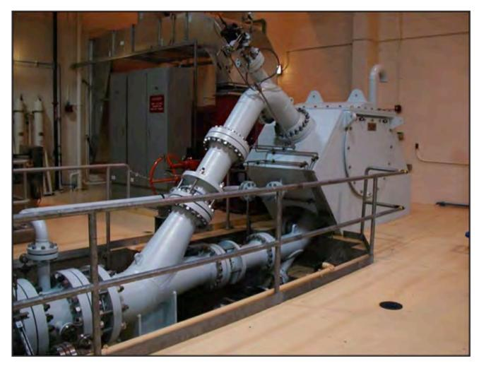
The Lakewood hydroelectric turbine and generator followed on the heels of the Lakewood Pipeline reconstruction. *Photo courtesy City of Boulder*
