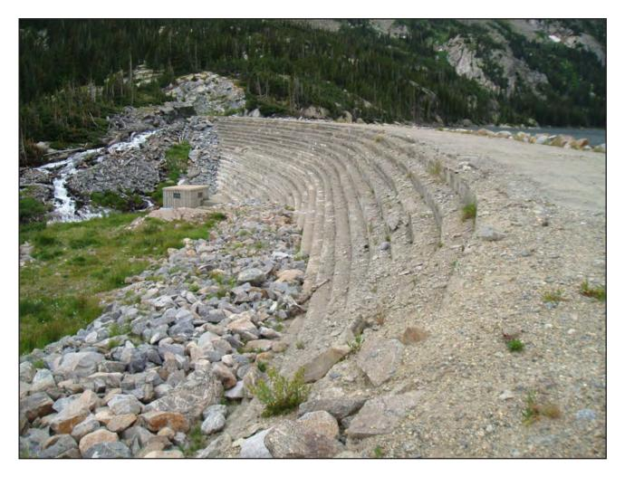
In 1989, roller-compacted concrete was installed on the downstream face of Goose Lake. *Photo courtesy City of Boulder*
