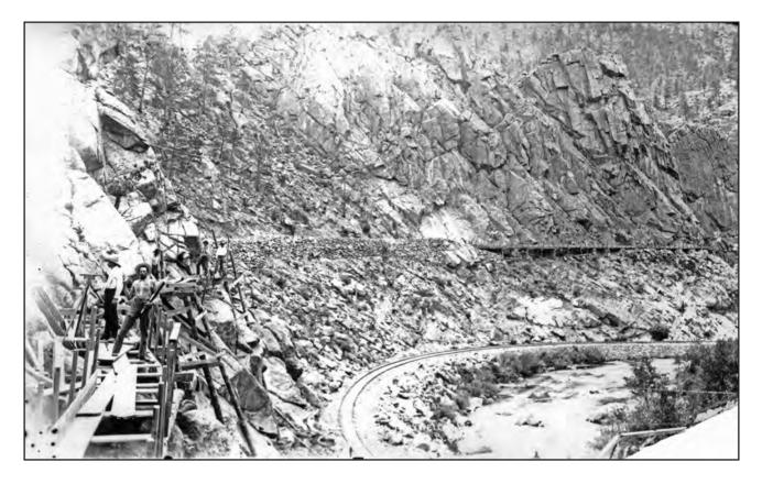
Laborers are shown, in 1888, constructing the wooden flume for the Silver Lake Ditch in Boulder Canyon. The line of the narrow gauge railroad (then the Greeley, Salt Lake & Pacific) is visible between the flume and Boulder Creek. *Carnegie Branch Library for Local History, Boulder (511-2-1 #1)*
