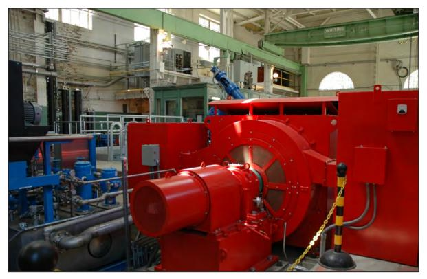
Above, a new generator and turbine, installed in the Boulder Hydro Plant, in 2012, replaced "Unit B"—one of two units dating from 1936. While keeping up with the latest technologies, the future of Boulder's waterworks also builds on its past. The photo, below, of the Boulder Canyon Hydro Plant was taken in 2013. Pettem photos , 2013
